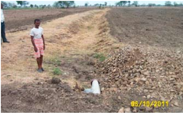
Installed underground pipeline with loose boulder structure in drainage line
