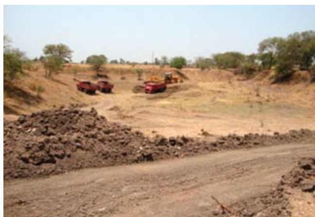
Shaping and deepening of excavated portion
