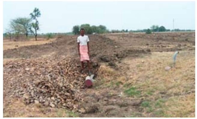
Installed underground pipeline with loose boulder structure in drainage line
