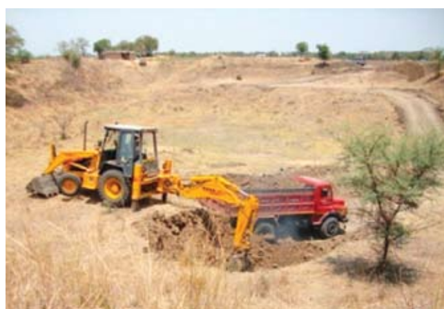
Shaping and deepening of excavated portion
